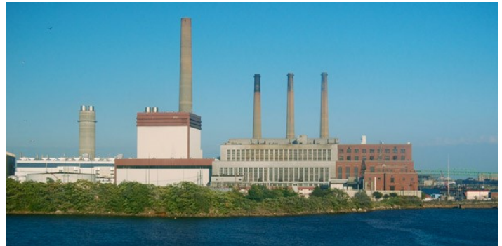
Mystic Generating Station
